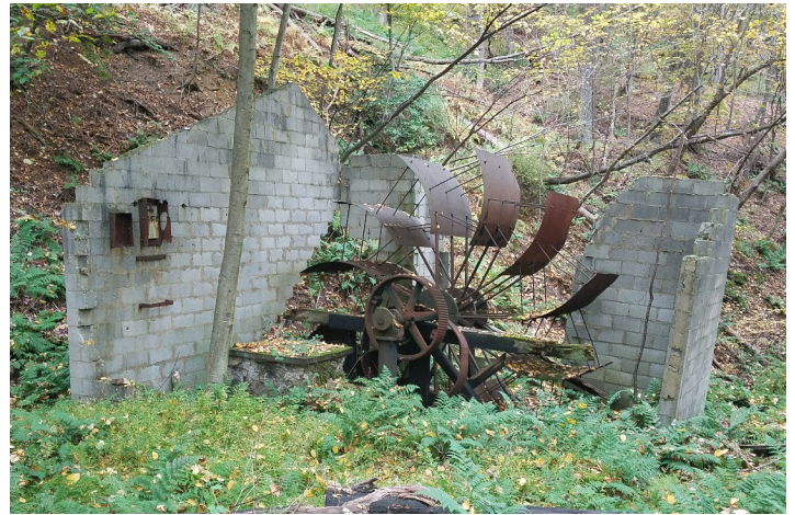
Another view of the fan house showing the cinder block walls and the large intact fan.
