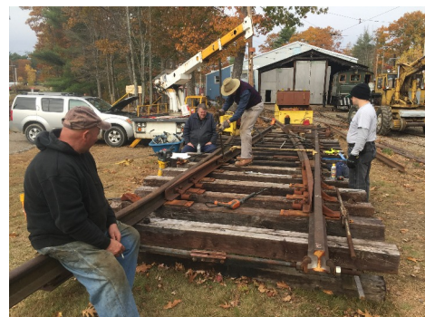
Once the crane has done the heavy lifting, there's only room for one person to tighten the point bolts.
