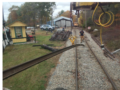
Rails longer than 39 feet were introduced more than 100 years ago. This 70 foot length of 70 lb/yard rail is flexible, but not so much that it can't be gotten off the ground by a Pettibone Speed Swing.
