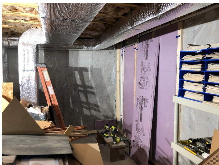
Insulation installation against the basement foundation walls
