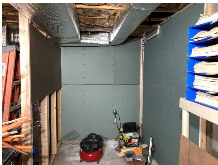
Drywall installed over the insulation
